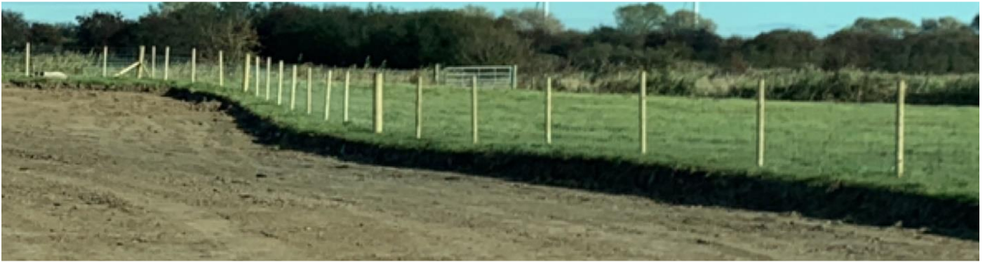
Figure 1.2: Example of post and wire fencing
